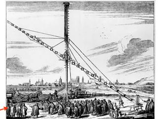
Woodcut illustration of a 46 m (150 ft) focal length Keplerian astronomical refracting telescope built by Johannes Hevelius
